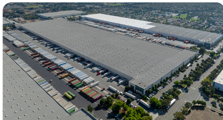
10681 Production Avenue, Fontana, CA
