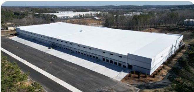
3945 Gilbert Road, Atlanta, Georgia
