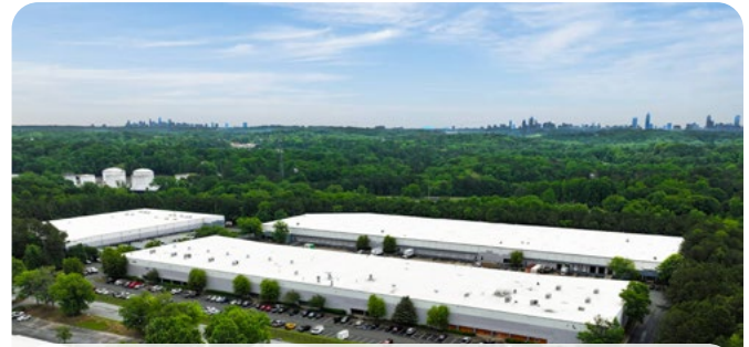
3655 Atlanta Industrial Drive, NW, Atlanta, Georgia
